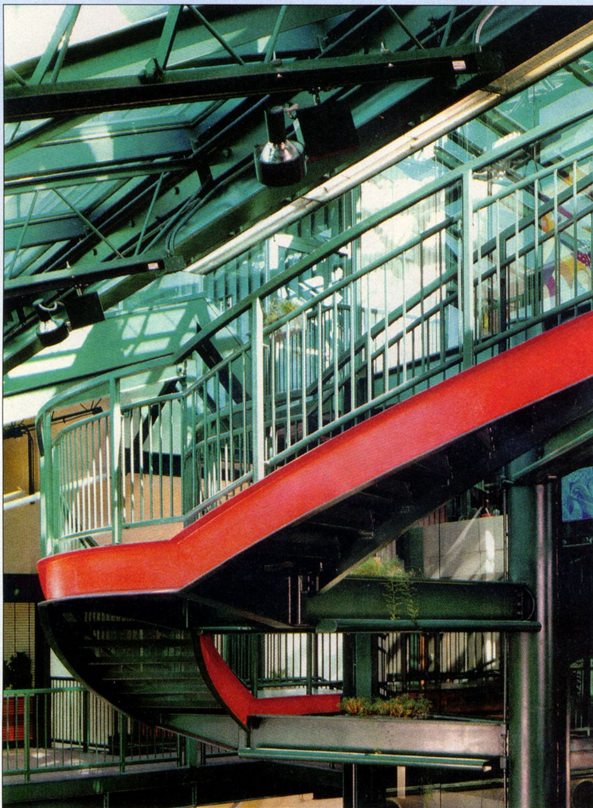
Steel “branches” extend from the central pipe (or trunk) to support the stairs.
