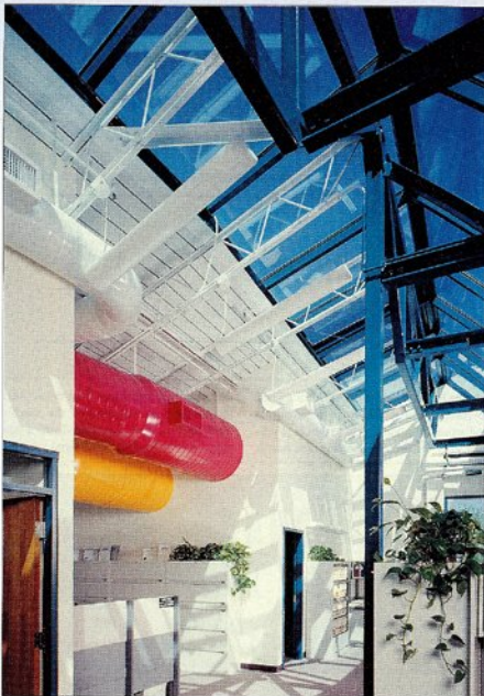
The exposed mechanical ducts and steel joists result in a light, airy interior office space.
