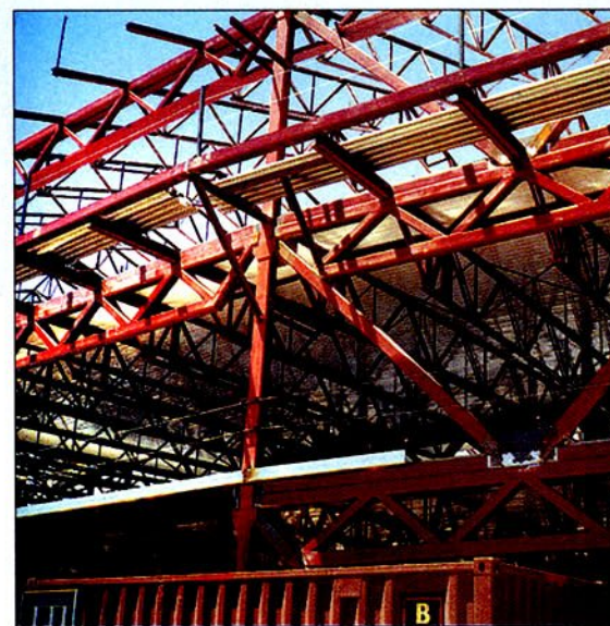
An inverted chevron braced frame is blended into a typical girder truss.
