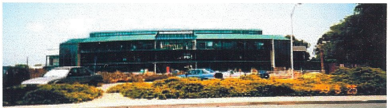
Front view of Pittsburgh Civic Center.
